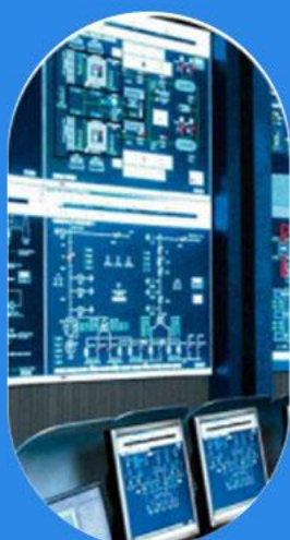
industrial control system
